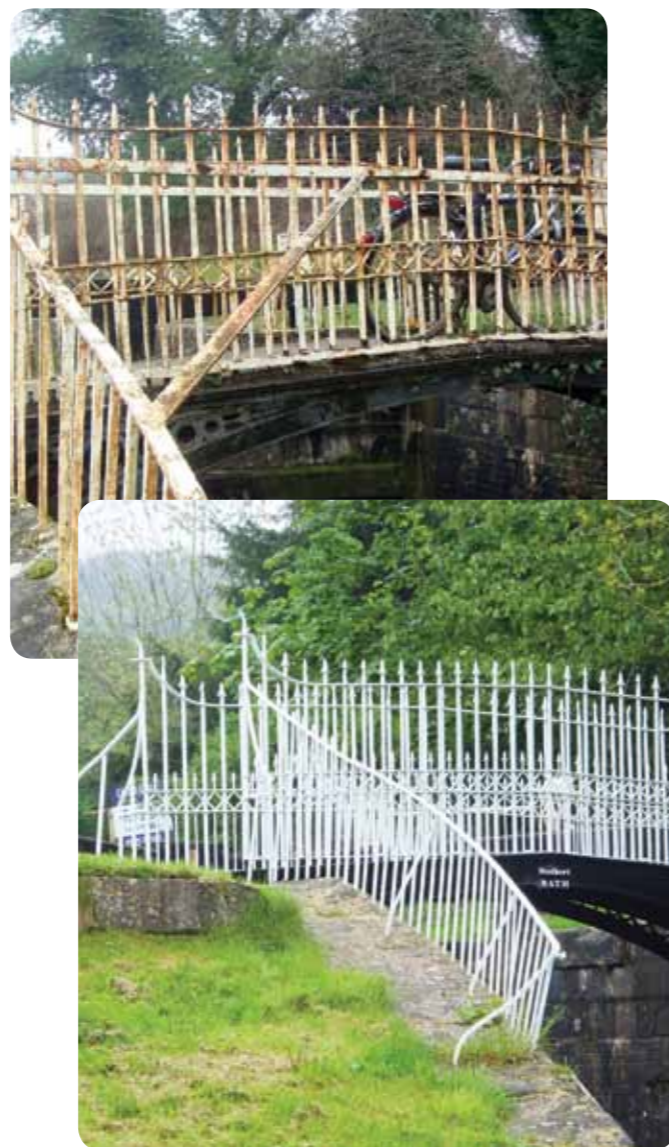
Stothert canal bridge, before and after restoration
